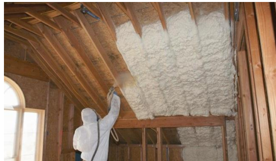
SPRAY FOAM INSULATION
