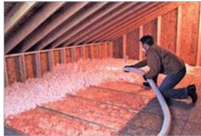
FIBERGLASS LOOSE FILL INSULATION
