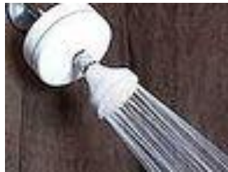
A mechanical shower timer installed on the shower arm
