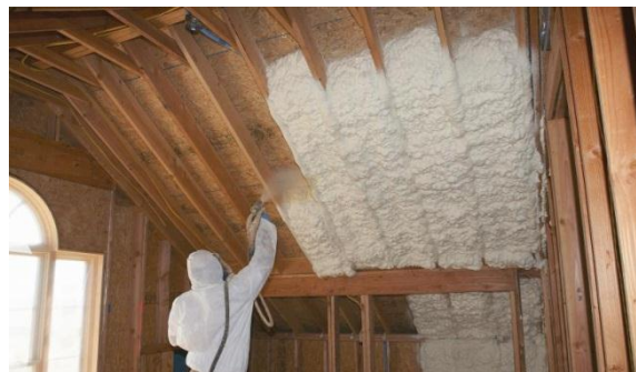
SPRAY FOAM INSULATION
